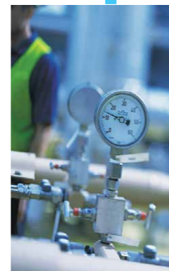
Valve Shutdown ( 30V DC 1A )
