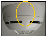
Picture 8 - Magnetic test area: correct position for magnet test
